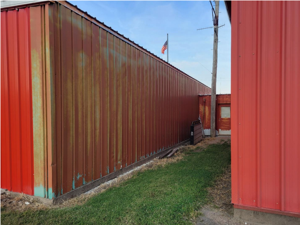
Photo 3: South Side of North Building
